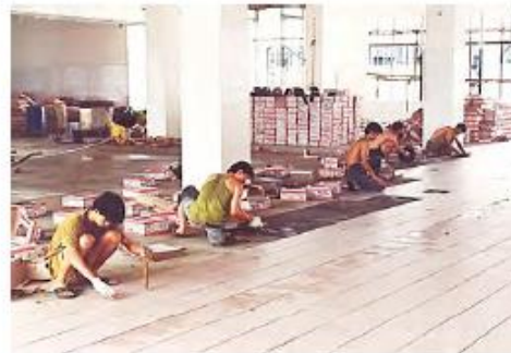
Tile Bonding & Waterproofing at Camel Nut Factory
