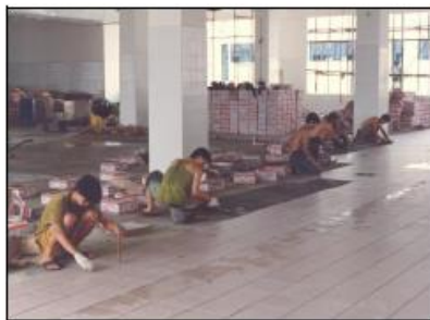
Tiling work by using W1 cement mortar Camel Nut Factory, Defu Lane 10. 2010 August
